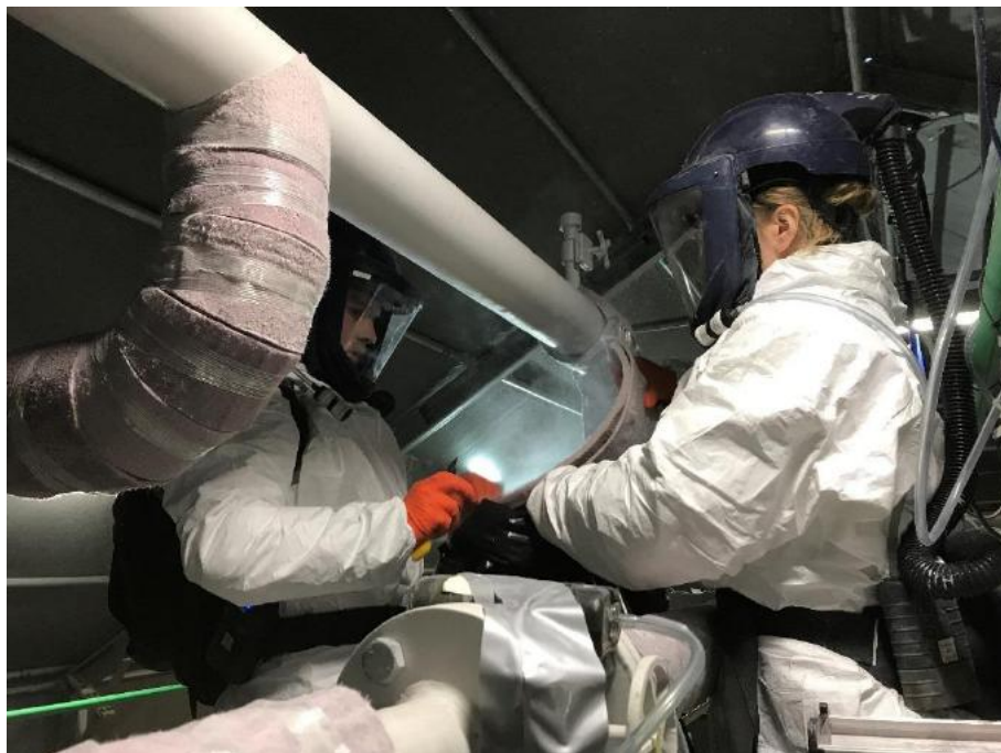
Figure 21: Removal of insulation
