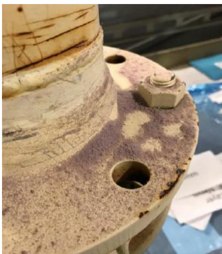
Figure 44: Settled dust on horizontal surface
