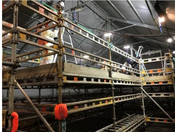
Figure 5: Overview of scaffolding
