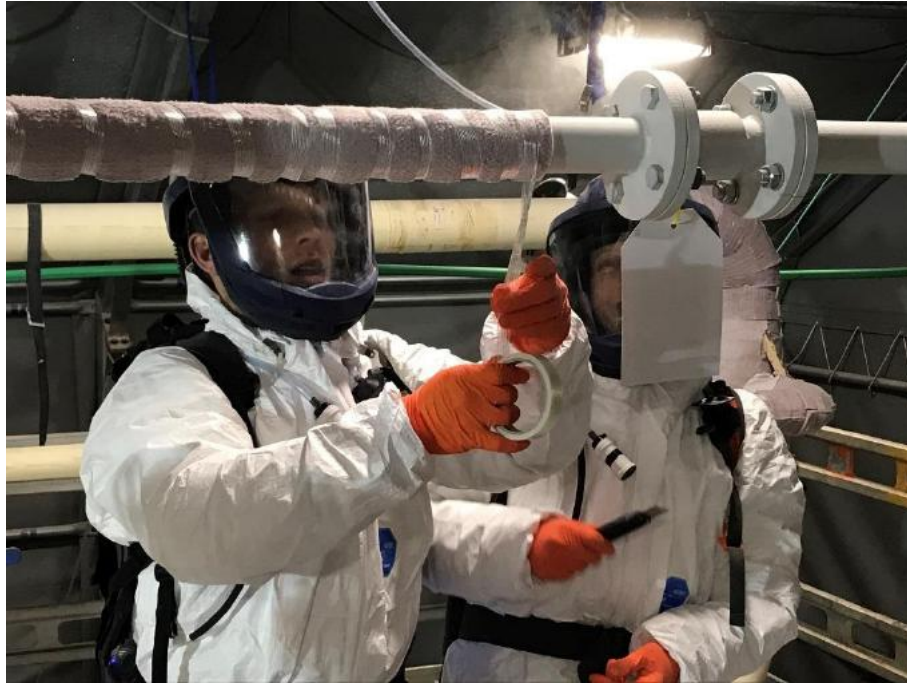
Figure 20: mounting insulation
