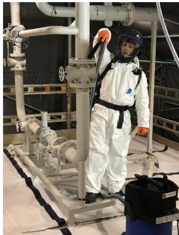
Figure 19: Cleaning by vacuuming
