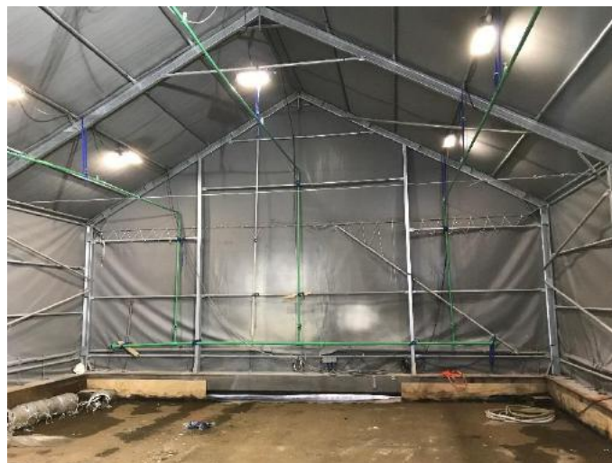
Figure 4: Inside rub hall prior to installation of scaffolding
