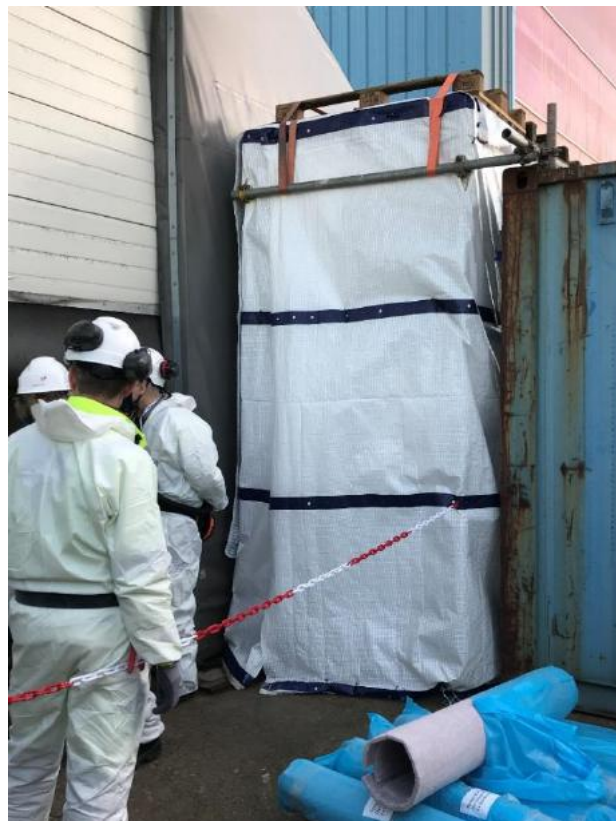
Figure 8: Cutting tent for insulation with entrance sluice
