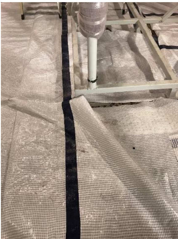
Figure 18: Scaffolding floor covered with tarpaulin
