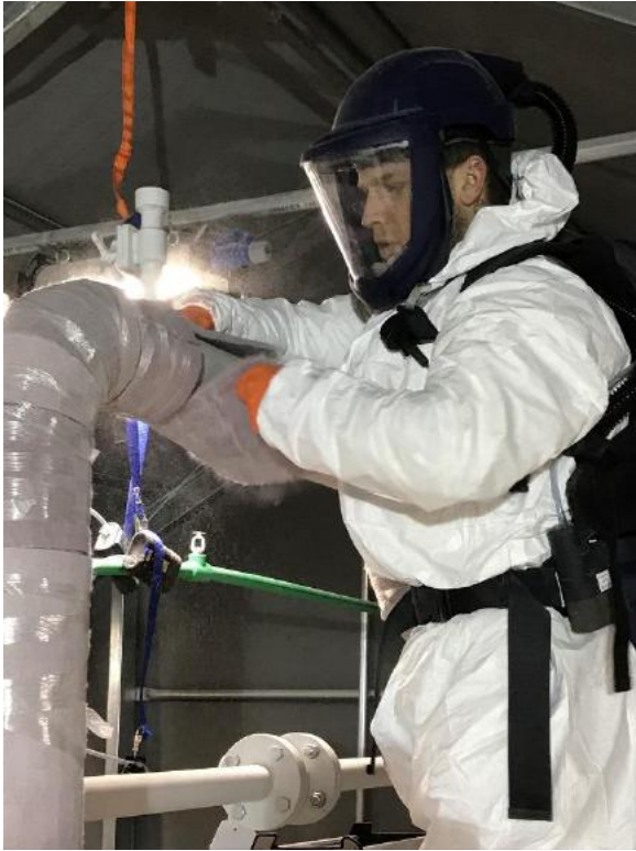
Figure 16: Insulator wearing respirator, disposable coverall, gloves
