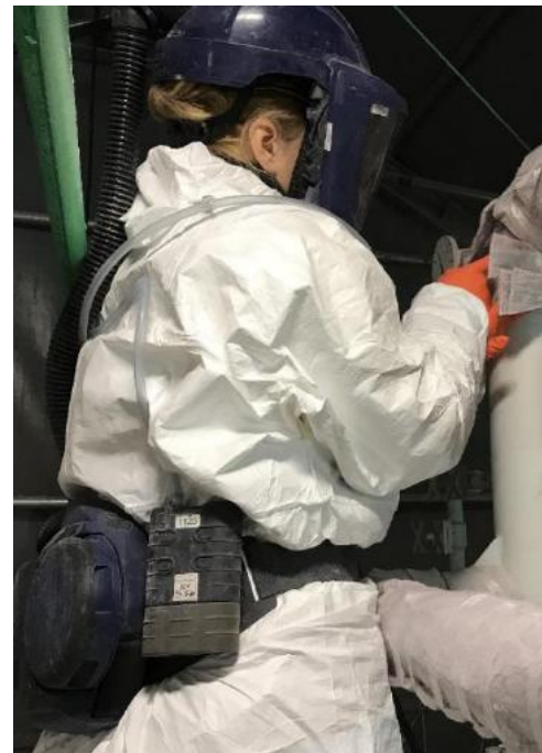
Figure 23: Pump mounted in insulators belt
